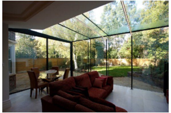
▲ A frameless glass box extension using low iron glass beams and fins with slim framed aluminium sliding doors as access to the garden.
