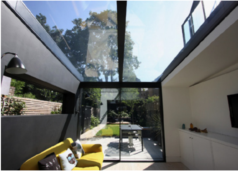
◀ This rear extension designed by HUT Architecture using slim framed aluminium sliding doors and structural glass roof above with minimal steel supports. To the side a frameless 'picture window' allows light in from the side.
