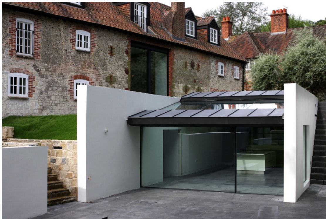
▲ A purpose built garden room within a still water feature to a residential garden in London. The room is fully glazed with fixed frameless glazing and slim framed aluminium sliding doors.
