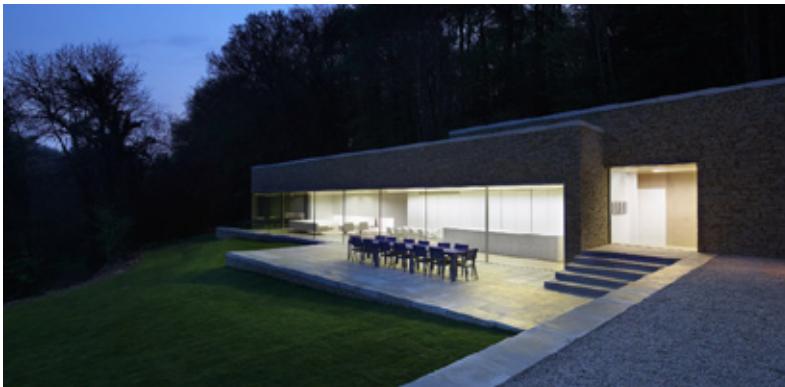
▲ Renovation and extension works designed by Found Associates. The main focus of the project was this linear extension with cantilevered roof. Beneath frameless structural glass runs down the full side of the living space with a single thin framed sliding doors as access to the garden areas.
