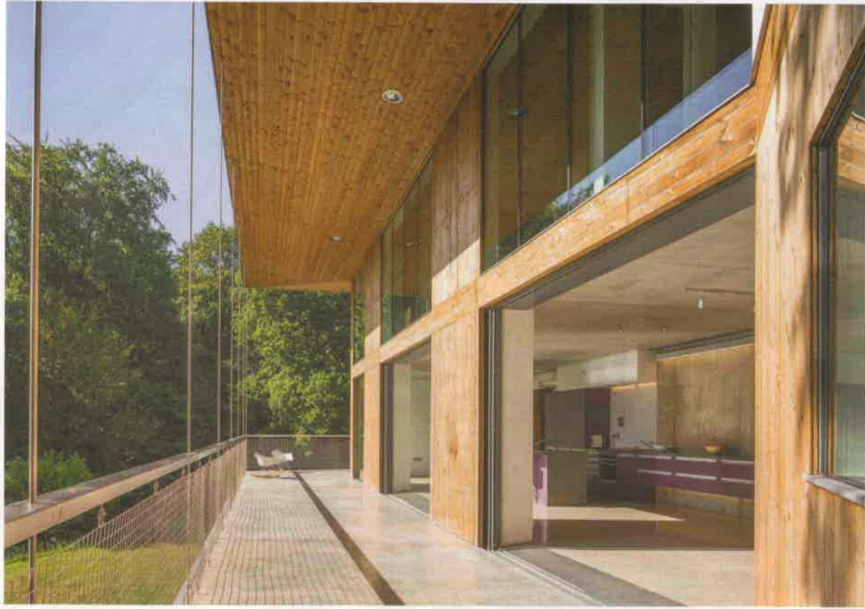
The west-facing terrace is suspended by stainless-steel cables.
