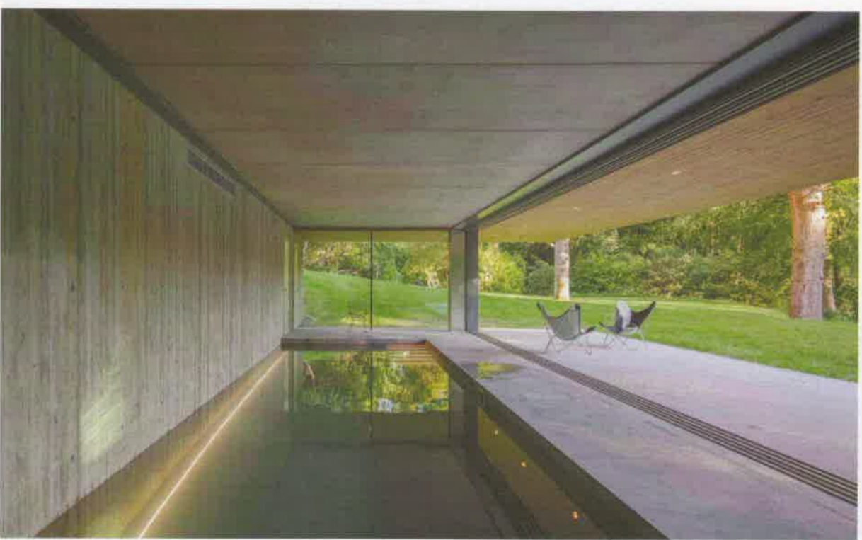
The lower ground level swimming pool.
