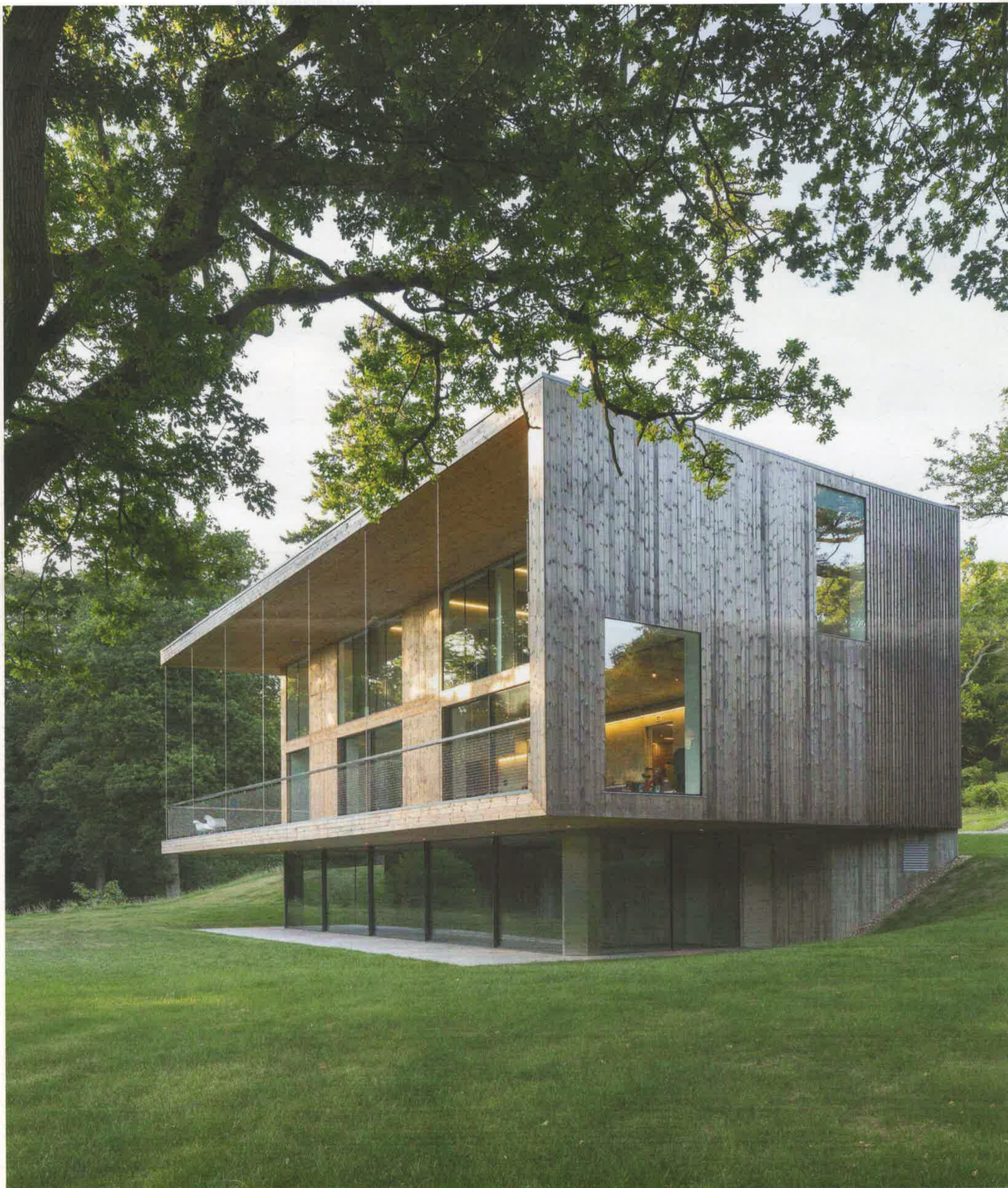
A Vierendeel truss enables the pool to open onto the landscape unobstructed.
