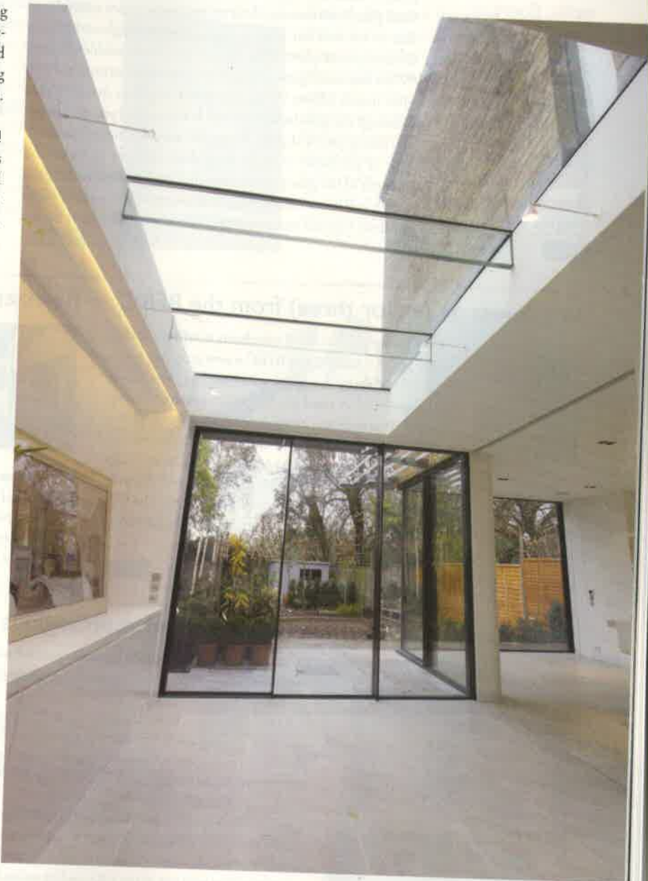
Frameless glass beams to glass roof
