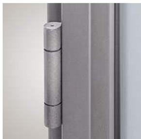
Three wing screw on hinge
