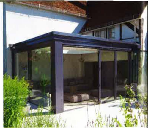
Right This glass-and-aluminium lean-to kitchen extension has automatic ventilation, which helps to keep the space comfortable on hot days. Similar structures by Apropos would cost around £40,000
